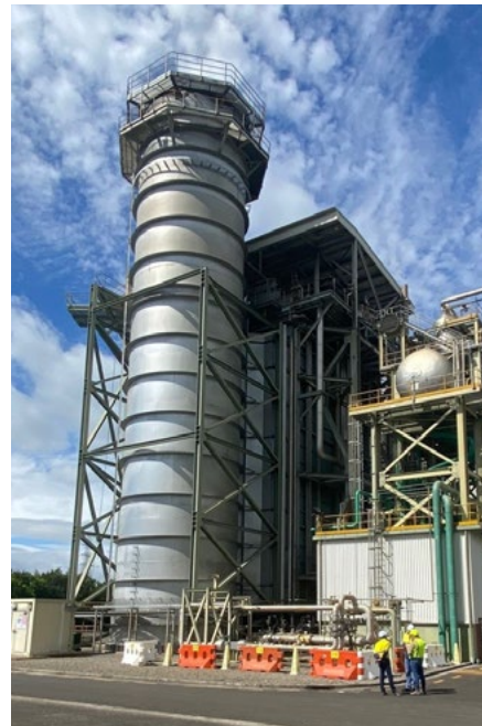
TCC's Heat Recovery Steam Generator at Stratford.
