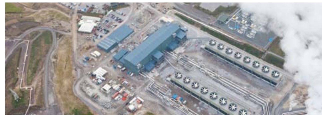
Aerial view of the Te Mihi power station. Photographer: Jeremy Bright.
